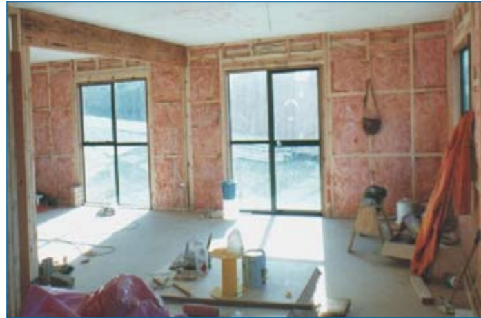
Inside of building refurbishment.
