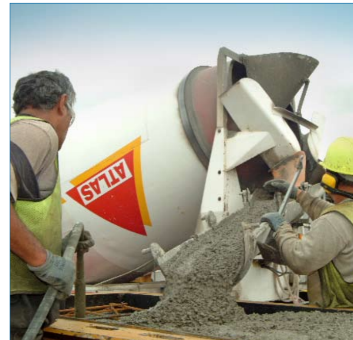
Pouring concrete in CIE precast yard.
